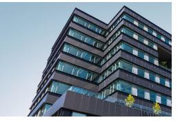
An integrated photovoltaic facade on a building from a project in Europe.
