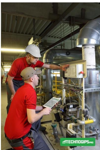
*Testing during the upgrade: Grenzebach experts checking a burner for proper function*
