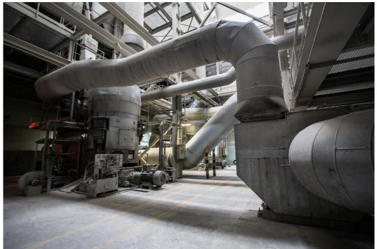
A 3D scanner allows the Grenzebach experts to precisely map existing equipment items and quickly and easily incorporate the new flash dryer system into the existing calcining plant.
